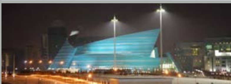
A DISTINCTIVE SAILING VESSEL OR ROSE SHAPE IS GIVEN TO THE BUILDING BY THE SLANTED SIDE WALLS.
