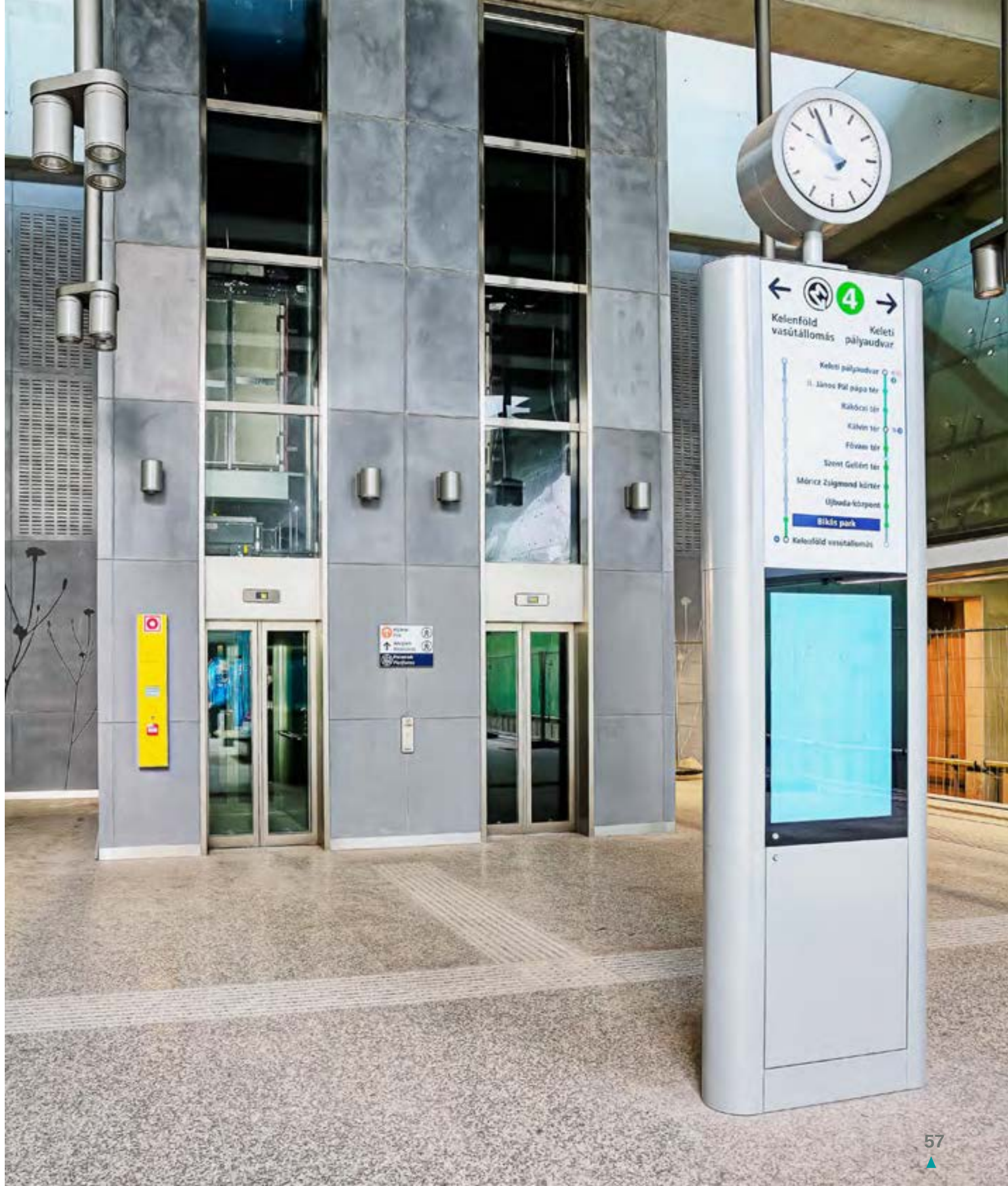
ELEVATORS INSTALLED AT BIKÁS PARK STATION
