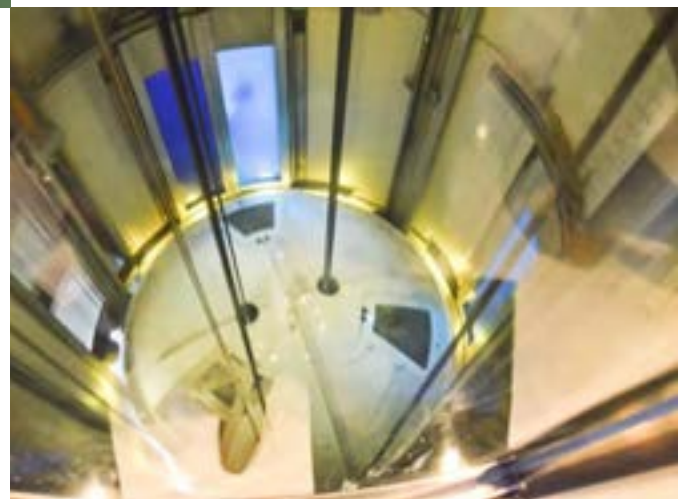
INTERNAL VIEW OF THE LIFT SHAFT
